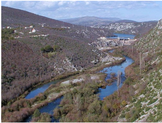
A dam on the Cetina river in Croatia
